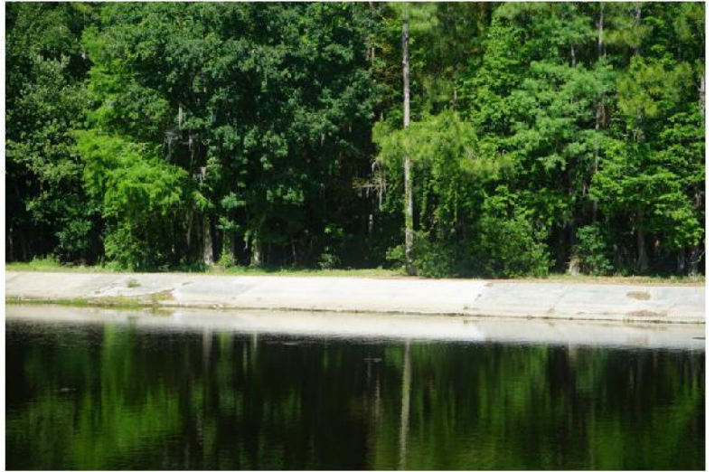
Weir wall section repaired
